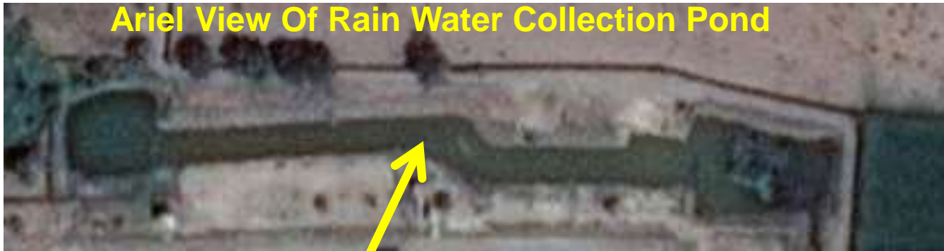
Ariel View Of Rain Water Collection Pond
